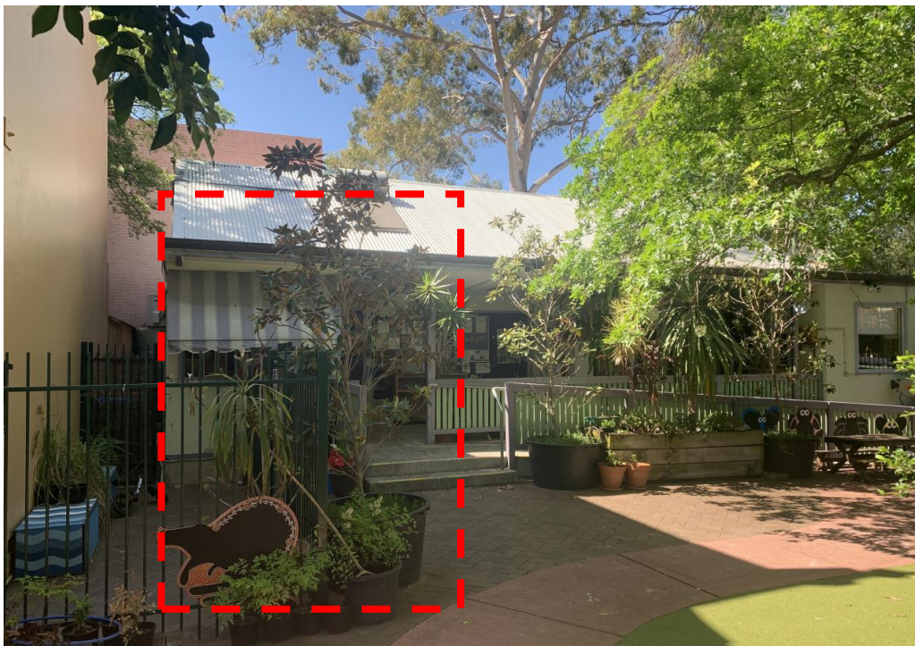
Figure 3: Looking south from within centres playground, at location of the proposed office extension highlighted in red.
